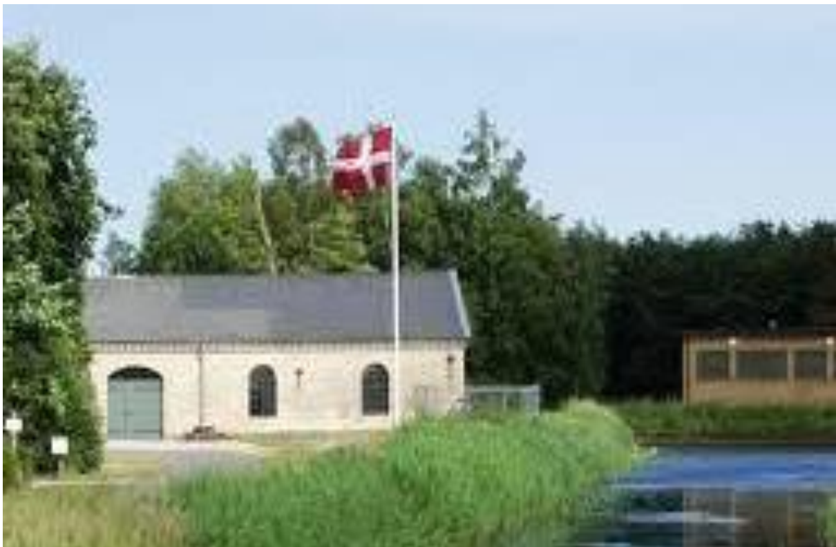
Marrebæk Pump Station
